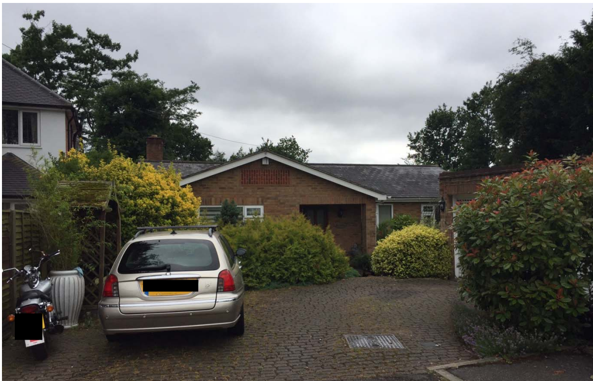
Existing front elevation of the subject property and detached garage, and the neighbouring property No.5a Crest View located to the left.
